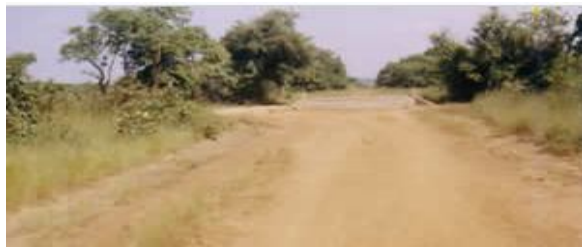
a. Section of Saboba-Wapuli road. Notice potholes and water at the far end.
