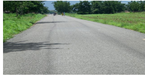
b. Intended road after upgrading
