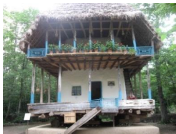
Figure 7. A traditional house faced to the south with openings only on the southern elevation
