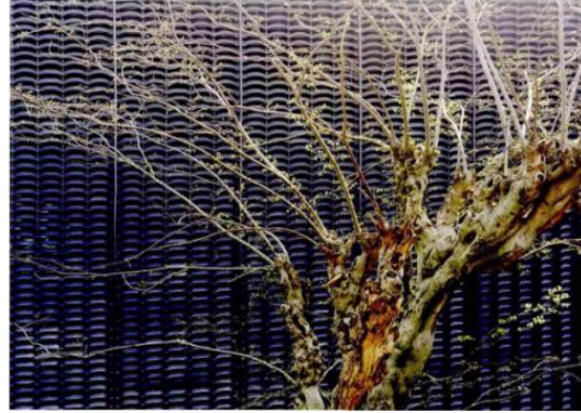
Figure 17 View the elevation from the courtyard
