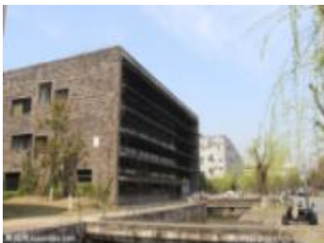
Figure 3 No.12 Xiangshan Campus, CAA
