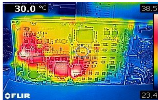
Figure 10: Thermal footprint of fully loaded LVPS unit after one hour of operations under ambient air conditions. Bright (hot) spots from left to right: buck MOSFET, main power transformer and 3.7 V rail Schottky rectifiers.
