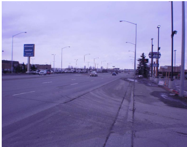
Figure 2. Dimond Boulevard looking towards C St from near intersection of Old Seward, 4/3/2011.
